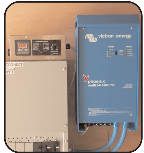
For “village power”, up to 15 inverters can be stacked for 3-phase operation.
